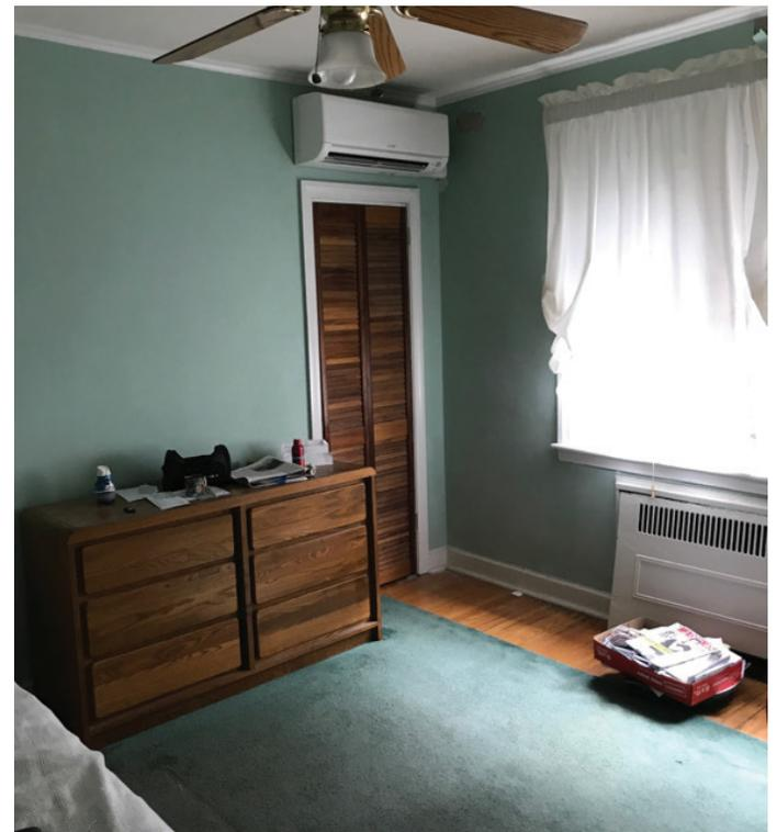
For this home, we designed a system that created five zones of comfort in the home, for the first floor living space and each bedroom. One outdoor unit like this one can service up to eight indoor units at a time, and each indoor unit can be operated independently, creating a separate zone of heating and air conditioning wherever it's located in the home.
